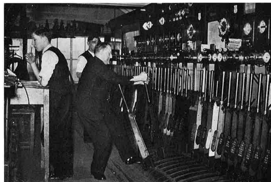
Interior of Selhurst Junction signal box
