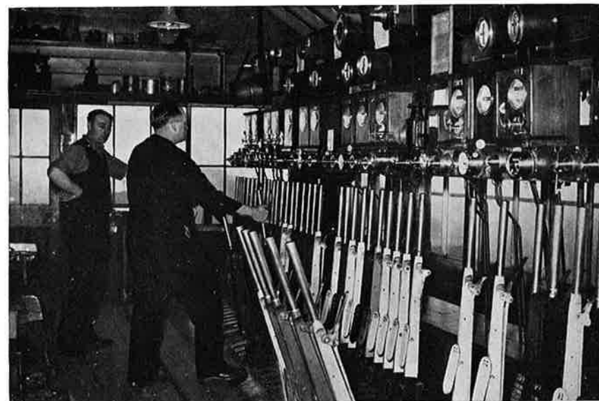
Interior of Norwood Fork Junction signal box
