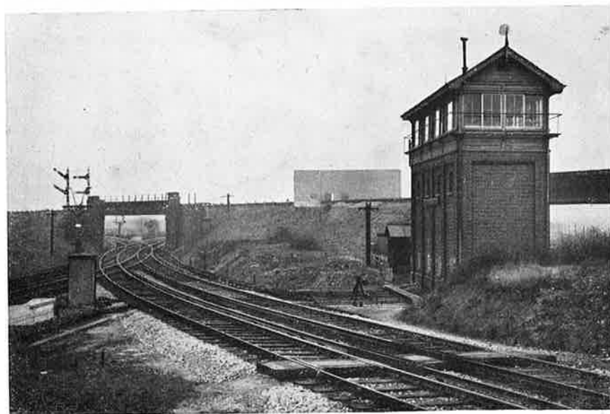
Gloucester Road signal box and flyover
